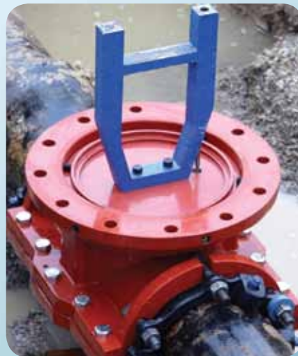
Internal equalization completion plug installed.
