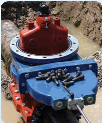
Low-profile bonnet used as line stop.
