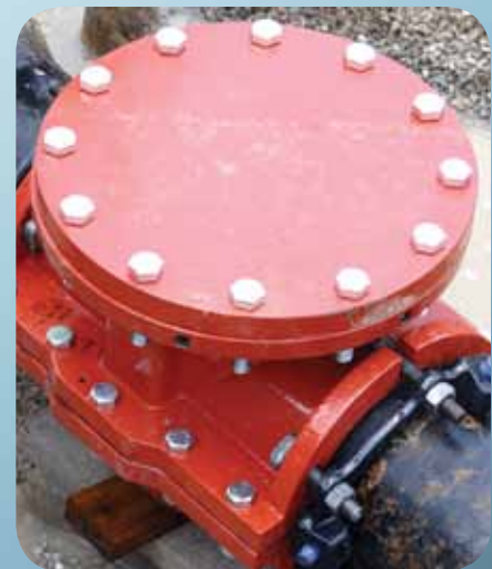
Blind flange installed.
